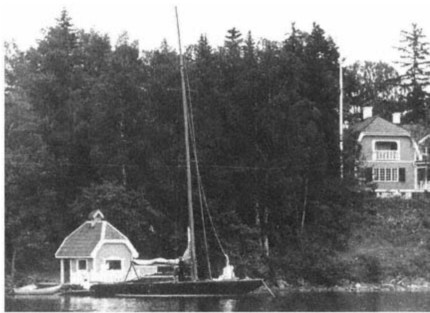
Siarö. In 1943 the trees were cleared and the studio was built up the hill from the boathouse, at the same elevation as the house.
